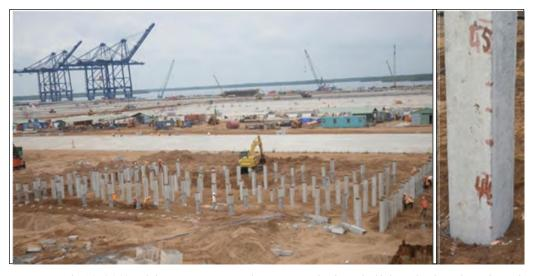
Fig. 10. View on Feb. 10, 2012, of the Maintenance Shop area with about half the piles lengthened (Authors' photo)
